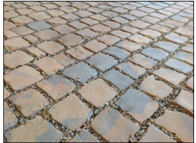
Imbedded grid structure links stones together into the Plaza mats.
